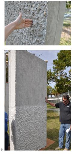
Back in Miami, the architects elaborated on the scratched texture of the Schaulager by chipping the 'out of form' surfaces, exposing the aggregate used in its construction but also giving the walls a texture more like the local Florida limestone of the region.
